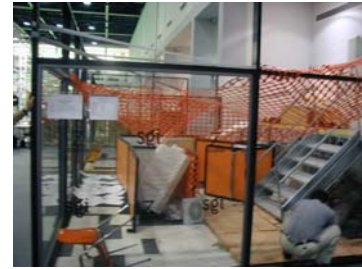
Figure 1: The Orange Arena
